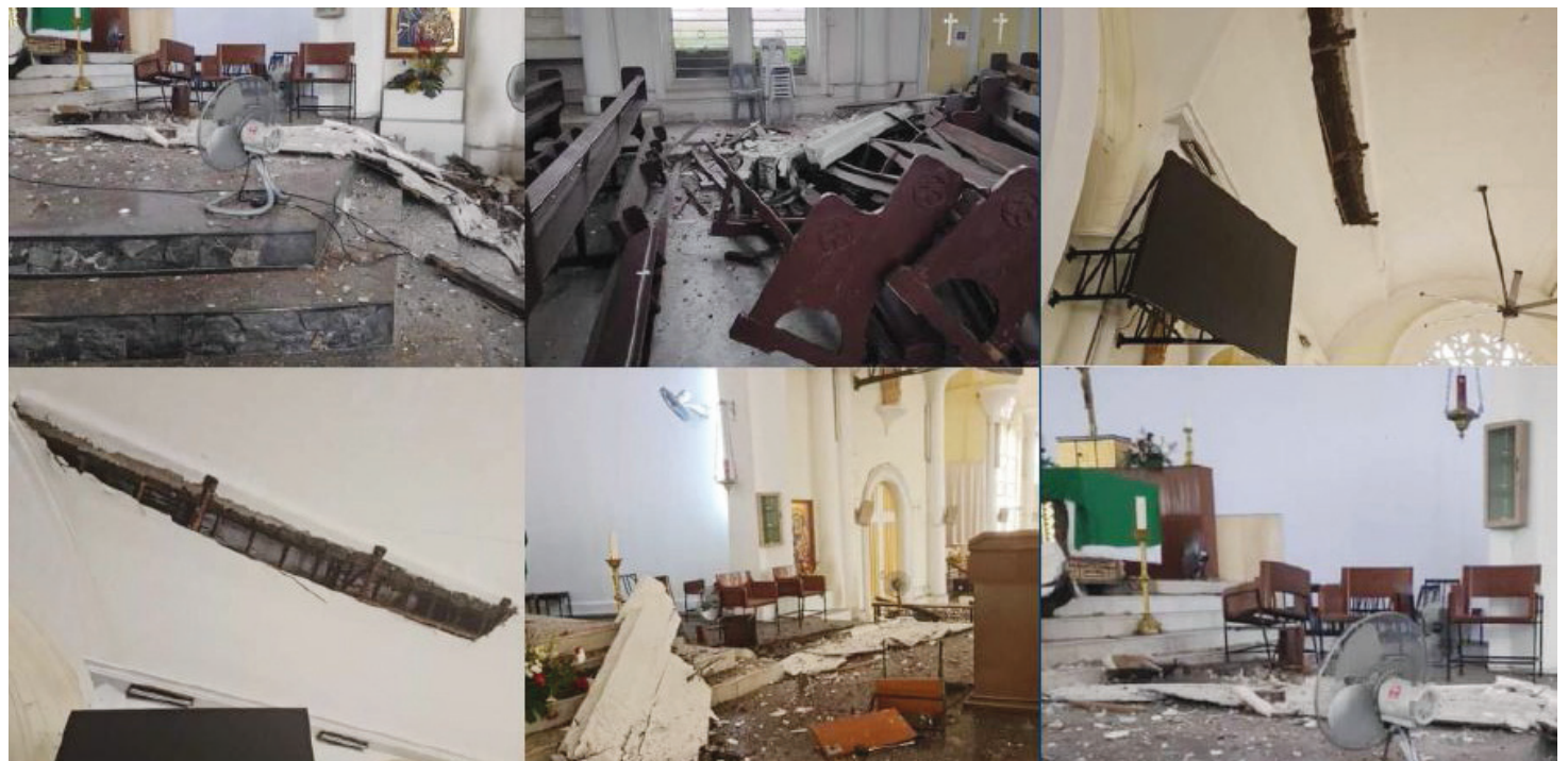
Part of the ceiling at St John’s Cathedral collapsed due to termite infestation. (Pic credit/Cathedral of St John the Evangelist Facebook)
